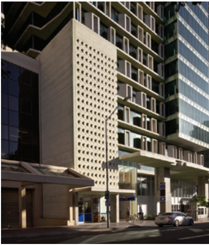
AM60 Building, Brisbane
