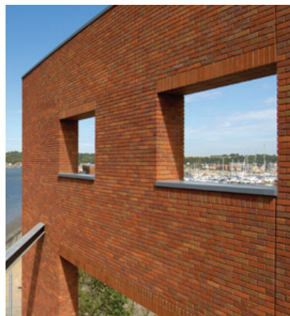
Soffit Support using LDB/S and Soffit Angle
