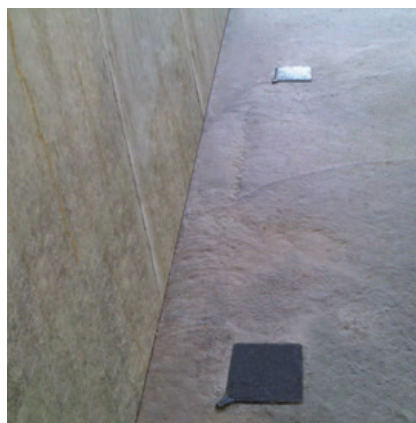
Void formers shown at Slab-to-Wall joint
