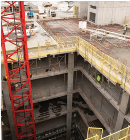
500 Lockable dowels were installed on the Emergency Care Centre in Aberdeen, UK
