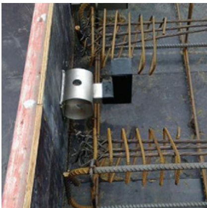
HLDQ-L30 Sleeve nailed to formwork
