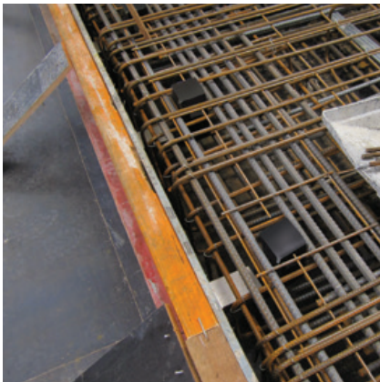
Reinforcement being located around ESDQ-L20 Sleeves
