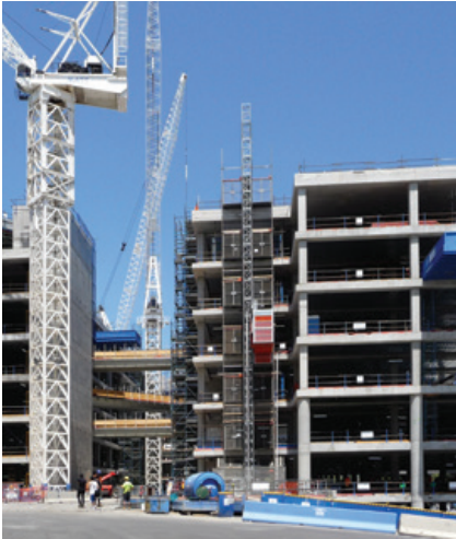
5,000 Lockable dowels were installed on the Royal Children's Hospital, Melbourne, VIC
