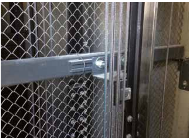
Framing channels and bolts
