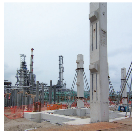
HALFEN HZA DYNAGRIP Channels cast vertically in columns to connect further components.
