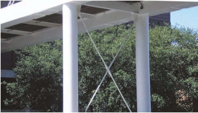
Cross-bracing with a cross coupler
